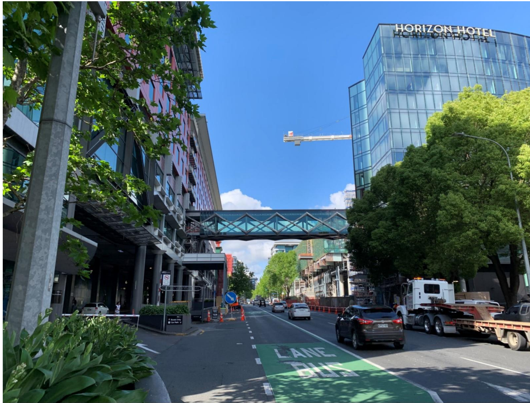
View from Hobson St – new linkway bridge
