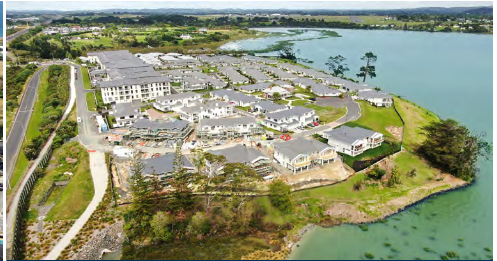
Summerset at Monterey Park (Hobsonville, Auckland)
