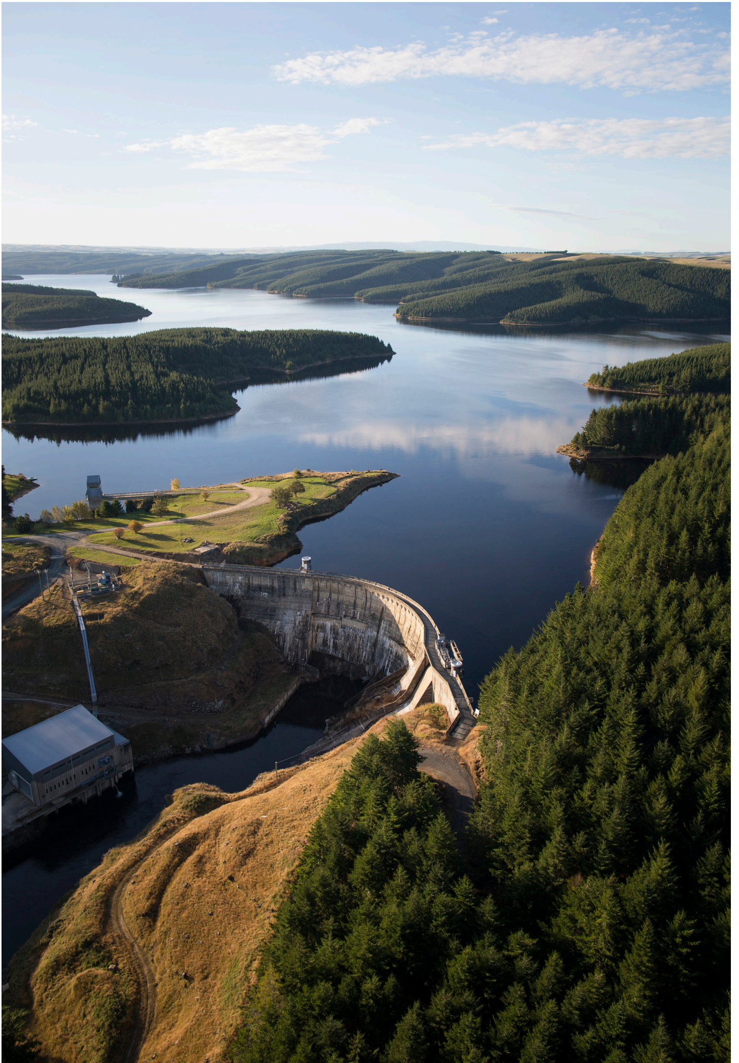
Waipori Power Station, Lake Mahinerangi
